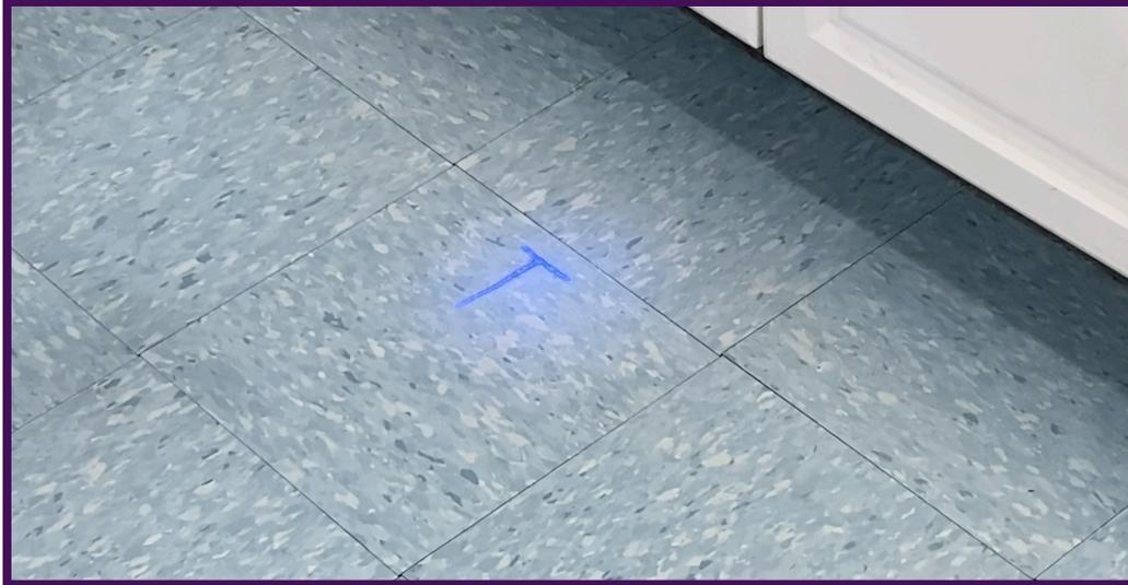
**2 UV lines added to floor one after the first coat and another after the second coat forming a 'T' on the floor. Checking the 'T' with a blacklight can show when finish starts wearing.**
