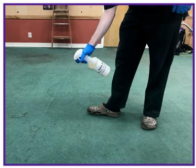
Step 5: Add 2 oz. per gallon Airx 80 from gallon container to extractor. We filled a bucket with water, then added Airx 80 and poured contents into tank of extractor.
